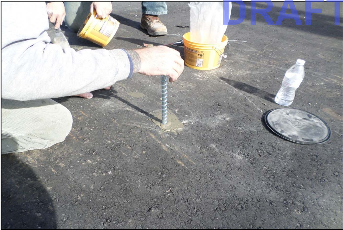
Photo 3 Anchor Modular Buildings installing a test anchor.
