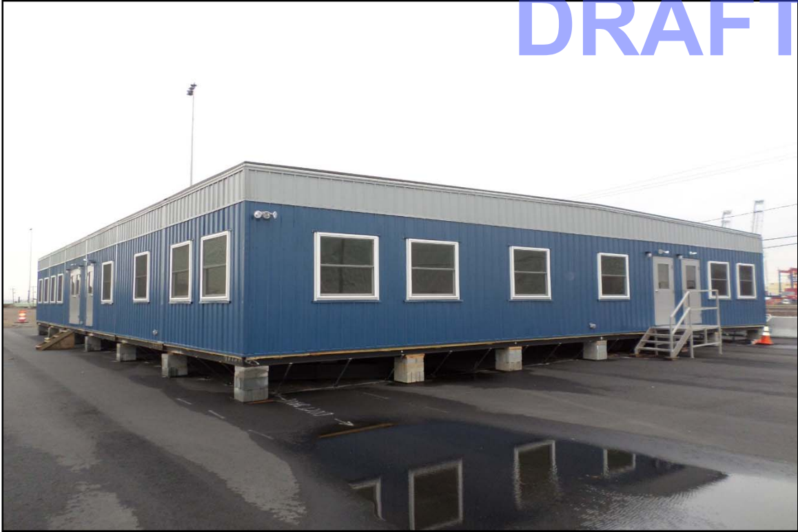
Photo 1 Overall view of the Greenville Yard ICTF Trailer, looking southeast.
